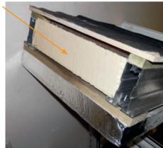
Once the plywood is fitted, cover the roof with breathing felt.
