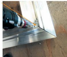
Fit facia board with poly pins on to timber batten Clip on gutter brackets and then fit gutter as it's easier to do so at this stage.
