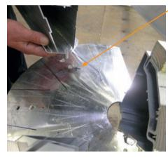
Secure Hips into Ridge End Plate using 13mm bolts supplied.
