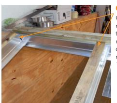
Once you have the rafters supporting the main body of the ridge start to slide all hip section on to ridge end plate using 13mm bolts supplied.
