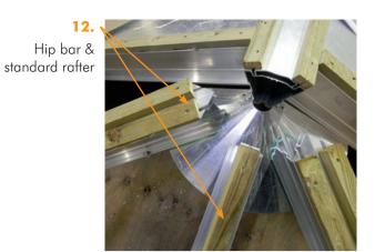
Cover the entire roof with 12mm plywood, fixing at the same time with either nails or screws onto hips & rafters using a minimum 35mm nail or screw (not supplied).
